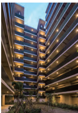
LED 開放廊下灯
